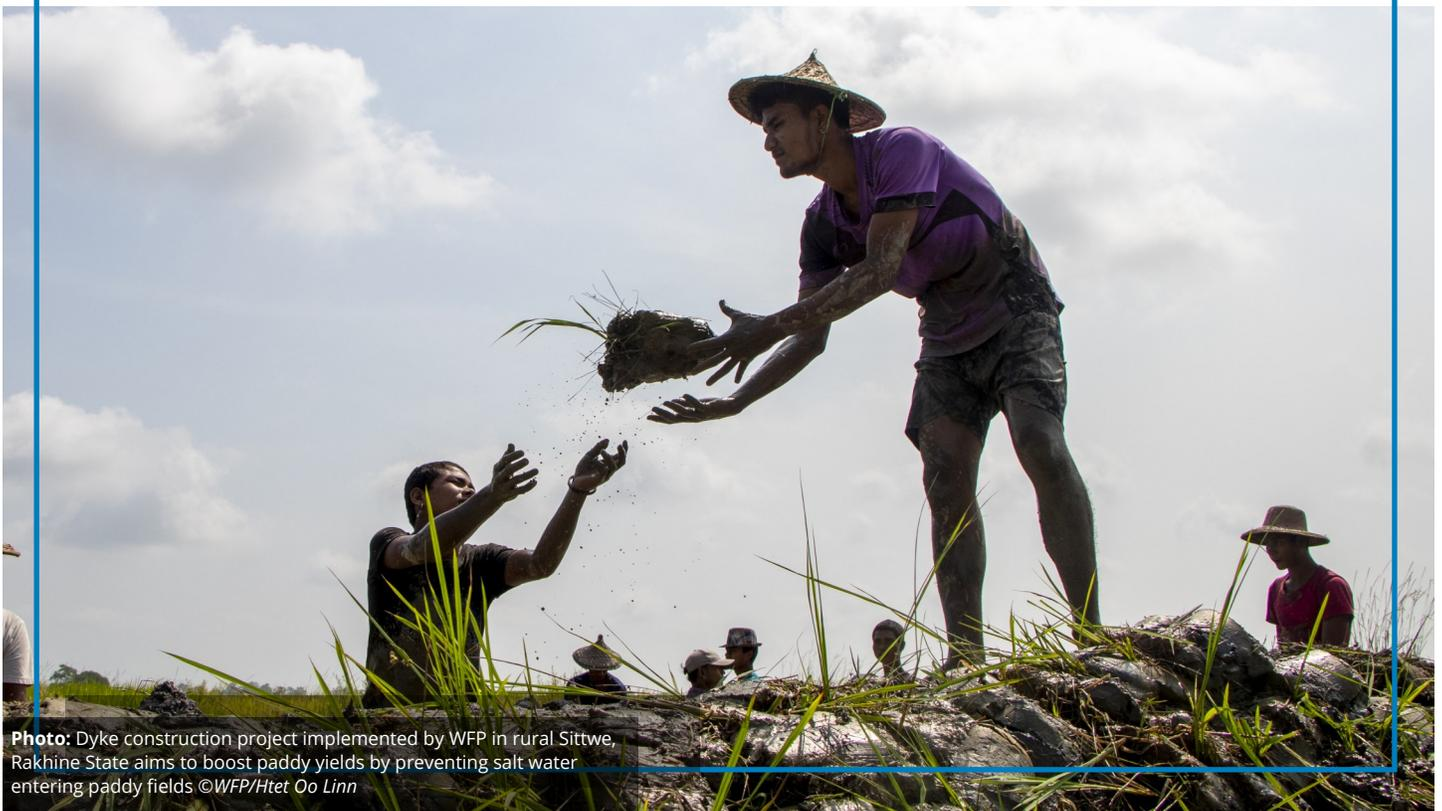
**Photo:** Dyke construction project implemented by WFP in rural Sittwe, Rakhine State aims to boost paddy yields by preventing salt water entering paddy fields ©WFP/Htet Oo Linn
