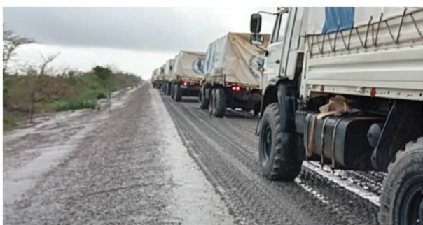
Trucks carrying humanitarian supplies traverse a newly rehabilitated stretch of the Bor-Ayod Road in Jonglei State. WFP has rehabilitated 240 kms of roads in South Sudan this year. Photo: WFP/ Allan Orimba
