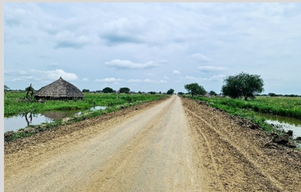
Photo: Completed road section between Baidit and Adwar (WFP)
