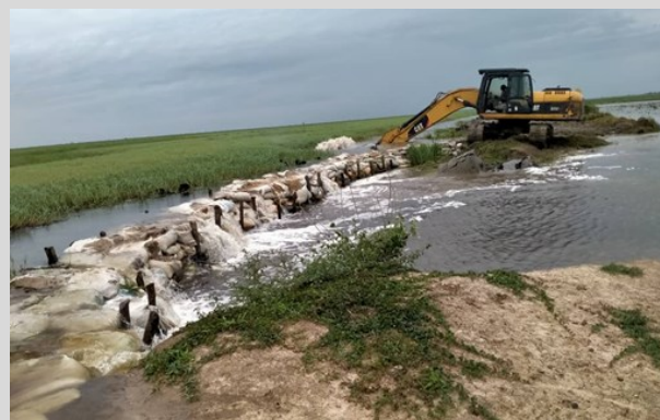
Photo: Progress of sealing breach points in Bor South (WFP)
